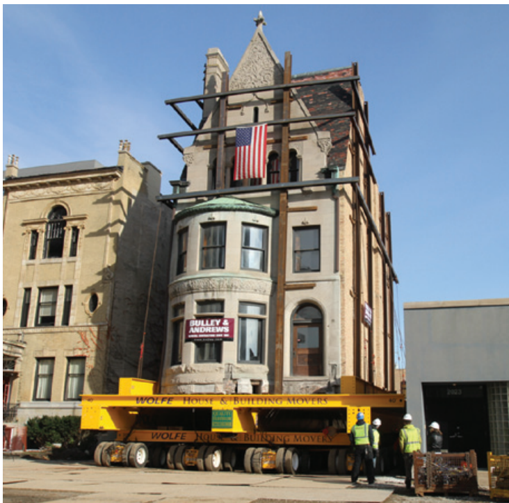
Bulley & Andrews (No. 222) relocated the landmark Harriett Rees House, Chicago, to allow for the development of an entertainment district. The 126-year-old, 762-ton building may be the heaviest-ever house removal in the U.S.
